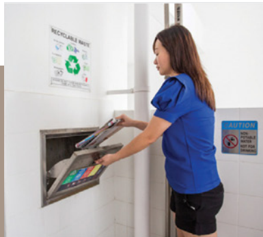
SEPARATE CHUTES FOR RECYCLABLE WASTE
